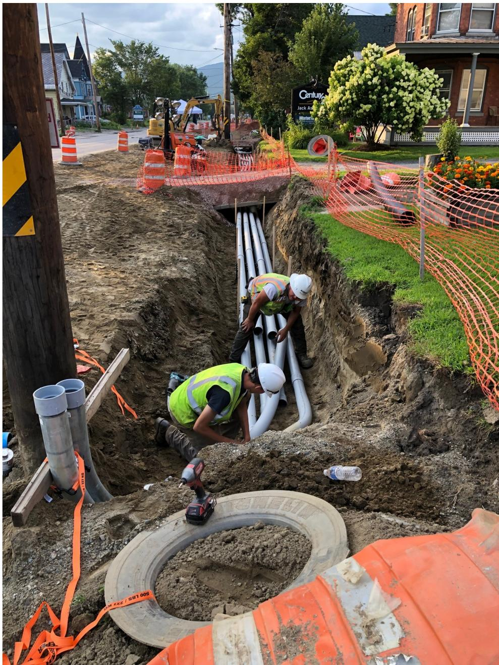
Long runs of conduit for underground electric and communication lines being installed under driveways and through parking areas.
